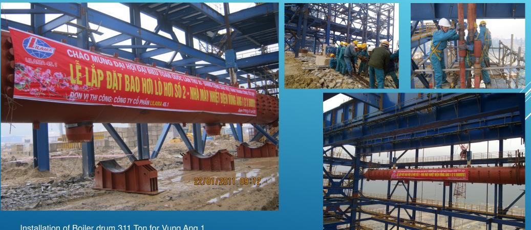
Installation of Boiler drum 311 Ton for Vung Ang 1 Thermal Power Plant
