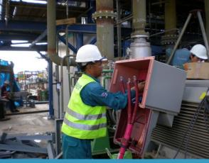
Connecting of medium voltage cable 6.6KV to switchboard
