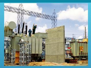
Installation of 01 Transformers 125 MVA, including 05 Route 220 KV and 07 Route 110 KV
