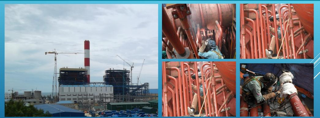
Installation of SH spay, SSH outet, RH outlet for Vung Ang 1 Thermal power plant
